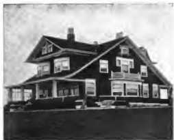
RESIDENCE OF JOHN C. THOMPSON, EAST LIVERPOOL
